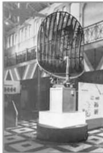
Early airport surveillance radar (Source: FAA)
